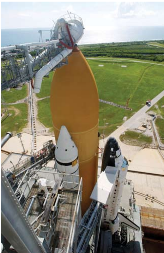
The gaseous oxygen vent hood (at top), known as the "beanie cap," is located on the end of the highest swingarm attached to the Fixed Service Structure.
